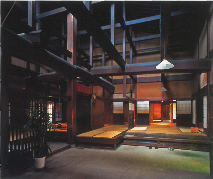
15 - Structural cage. Yoshijima House, Takayama, 1905.
